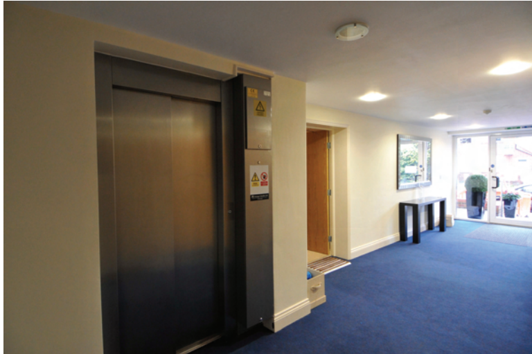
Picture 4.2 An accessible lift in a communal hallway
