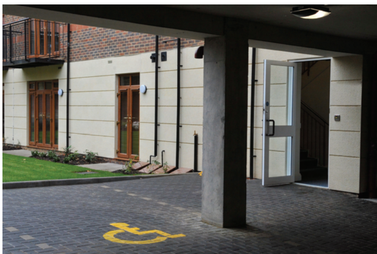
Picture 4.8 An accessible parking space & level approach
