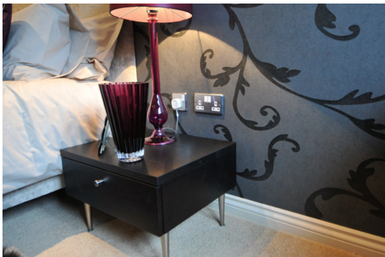
Picture 4.6 Electrical sockets 450mm above the floor
