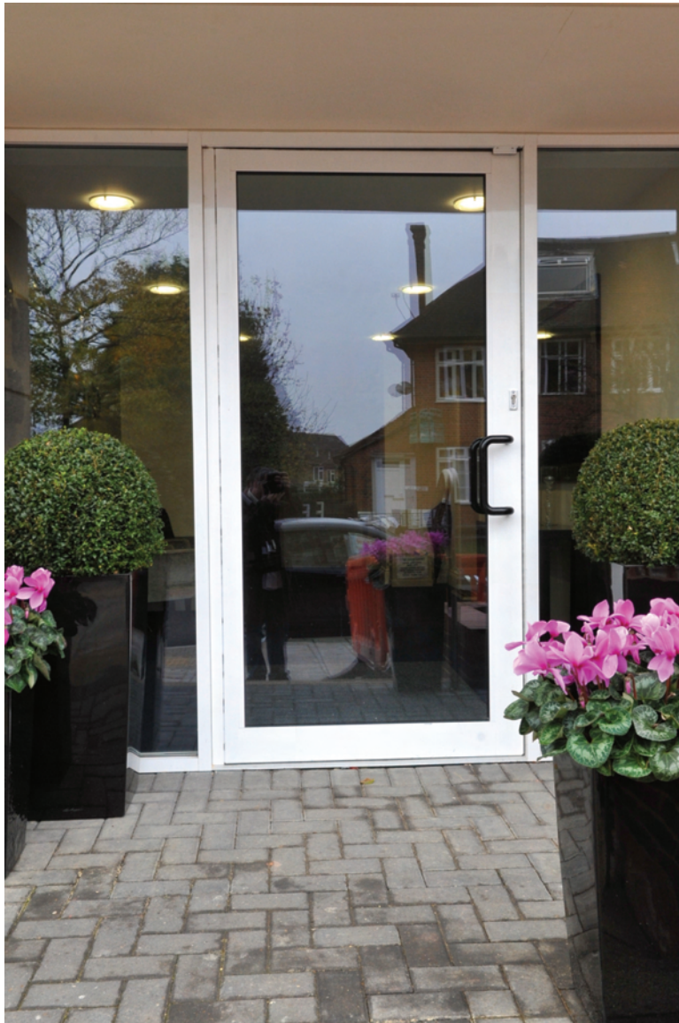
Picture 4.1 Covered entrance with level access
